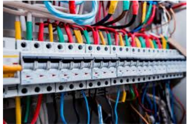
Figure 1: Electrical Panel the Electrical Panel Which Is Under Repair
