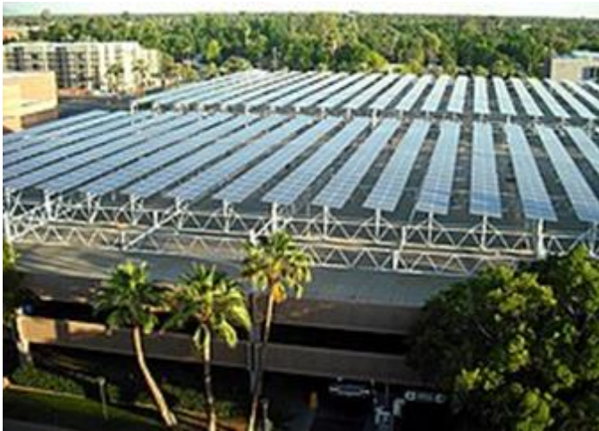
Figure 2: Solar Tracking Array
