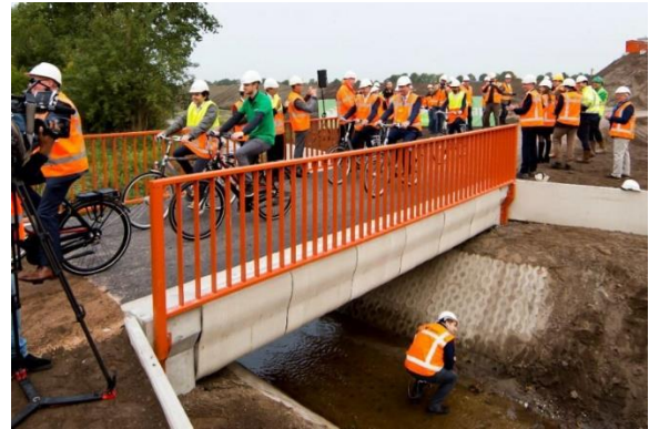
Figure 9: The first 3D printed bicycle bridge [45]
