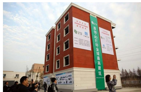
Figure 6: Multi-story buildings printed by WinSun [41]
