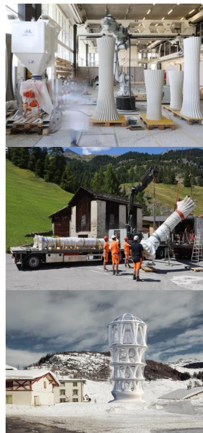
Figure 17: The photos are the printing process, assembly and design of Tor Alva, respectively [52]
