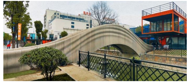
Figure 13: The world's longest 3D-printed concrete bridge [44]
