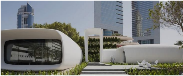
Figure 7: The first office in the world constructed with 3D printer technology (Office of the Future in Dubai) [43]
