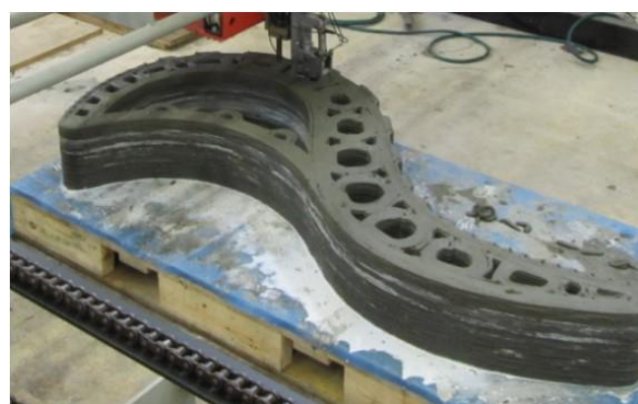
Figure 2: Concrete Printing Method [38]
