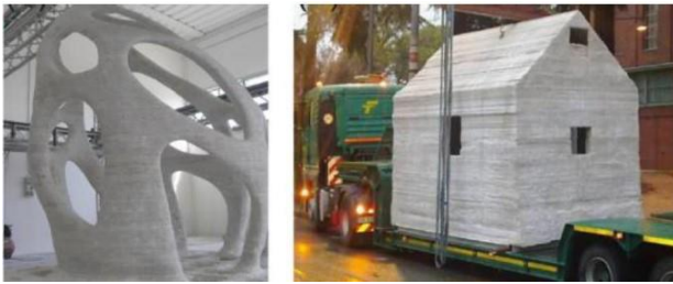
Figure 3: D-Shape Method by Enrico Dini [39]
