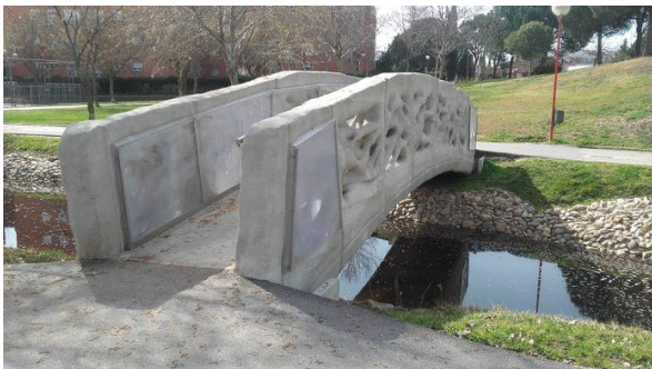
Figure 8: The world's first large-scale 3D-printed concrete pedestrian bridge [44]
