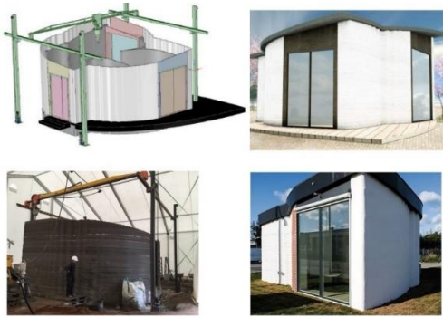
Figure 20: 3D printed house printed by 3D Printhuset in Denmark [61]
