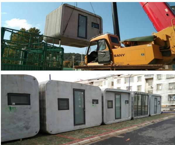
Figure 16: 3D printed isolation room in China [51]
