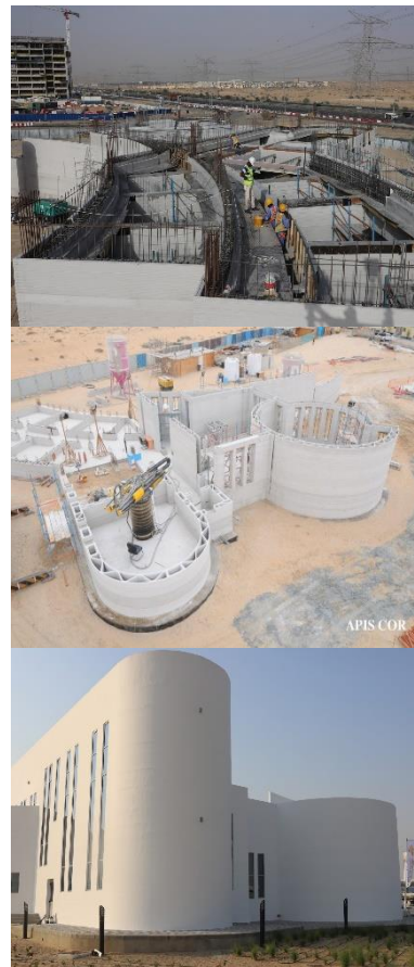
Figure 14: Dubai Municipality Office in the United Arab Emirates [10]
